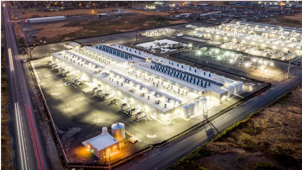
Figure 2. An Amazon data center in Umatilla County, Oregon, USA
