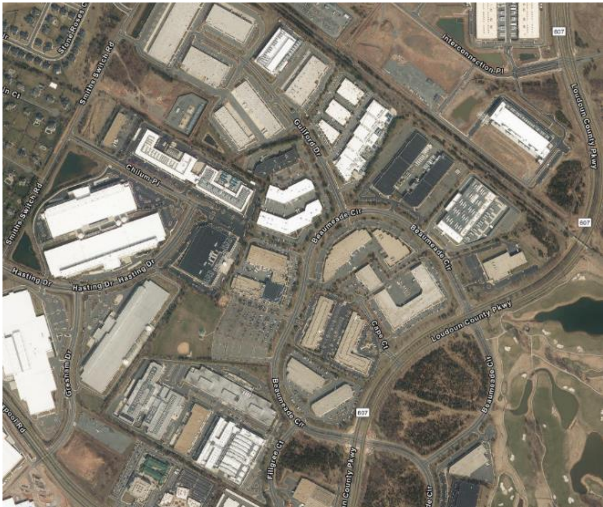
Figure 6. A cluster of data centers located in Northern Virginia, USA [8]
